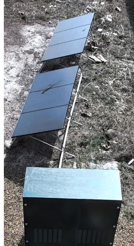
Solar panel to power the smart city cameras.
