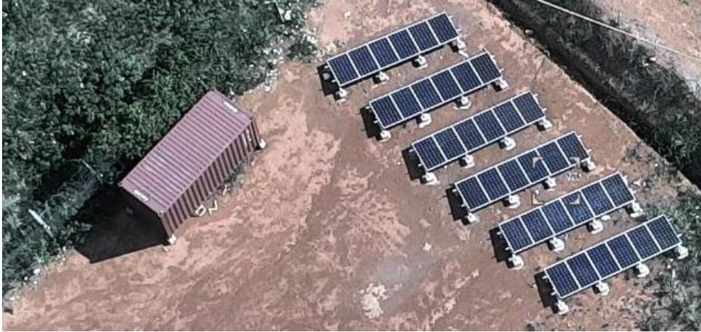
6KW Solar Farm to power the Camp Fidel our backbone transmission center
